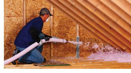
ProCat® Insulation is a loosefill fiberglas™ thermal insulation. It is designed for use exclusively with the ProCat® machine.
